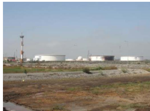
Figure 16. El Maule, Chile 2010 earthquake, ENAP Bio Bio Refinery. Earthquake directivity.
